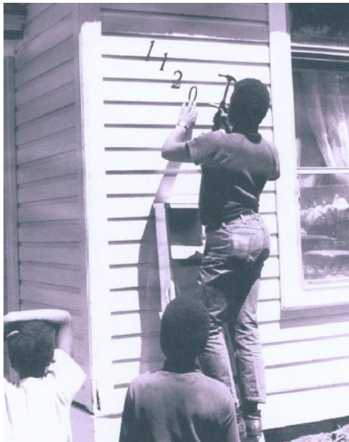
Figure 60. Men work on a house in River Street, 1970 (from the collection of John Bertram).
