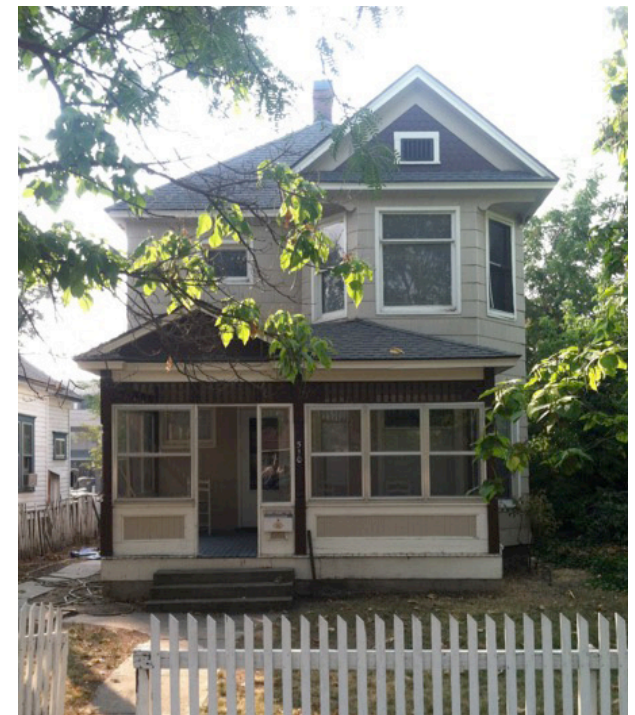
Figure 72. Refurbished house on S. 14th Street, 2014 (White).
