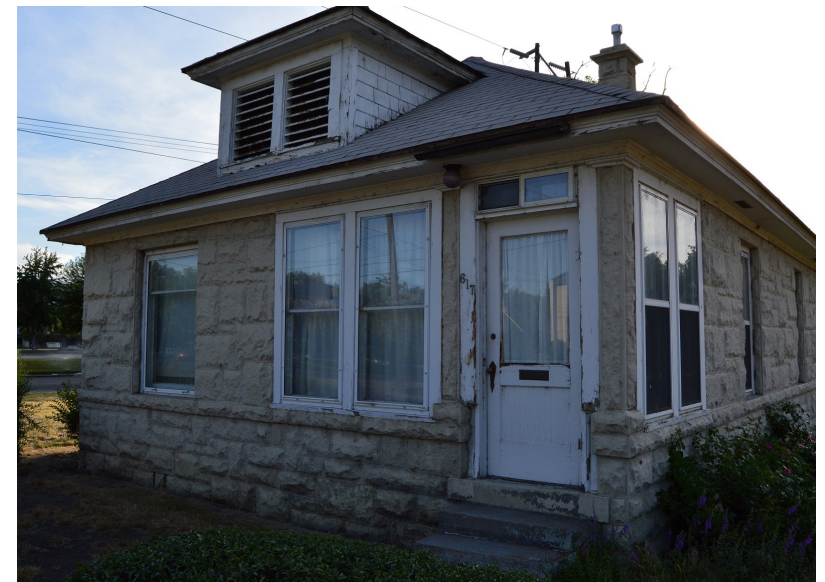
Figure 62. Dick Madry’s grandmother’s house is one of the few historical homes left in River Street, 2014 (White).
